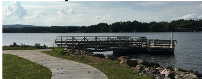
Accessible Fishing Pier – T dock
