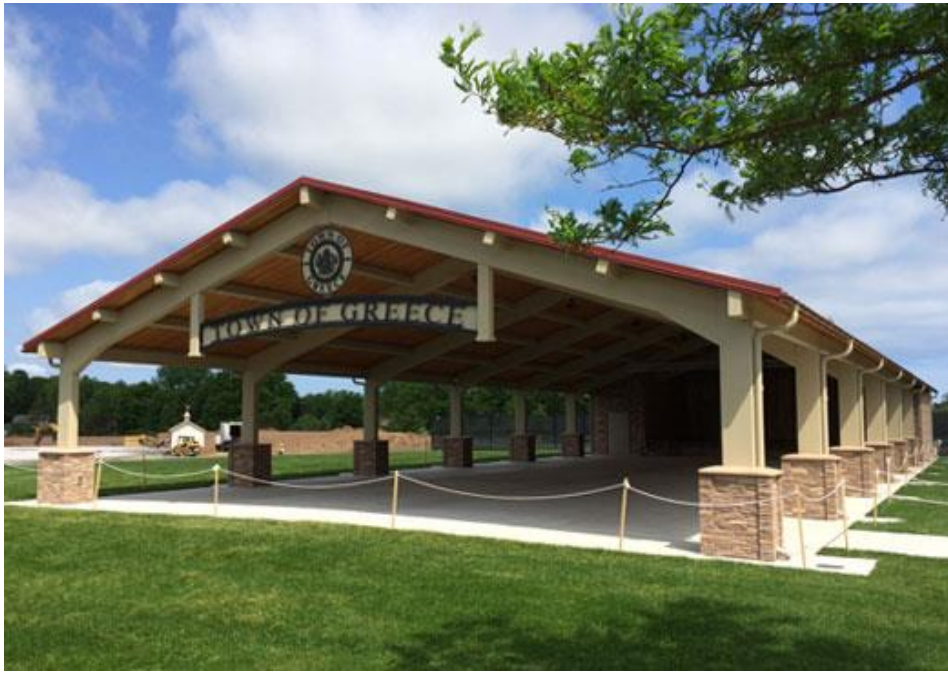
Large Pavilion with restrooms and kitchenette at the end
